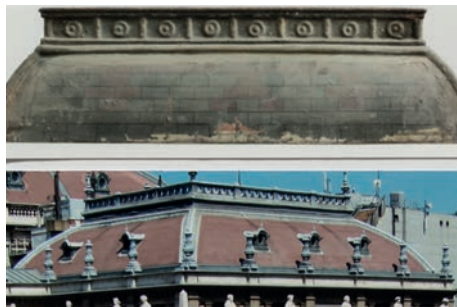
Fig. 6 a–b. Curved line roof ridge a) on the intermediate element and b) on the Hungarian State Opera
