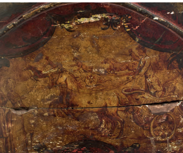
Fig. 25. Shell-shaped outbreak of the painted ground layer along the joints and its repair
