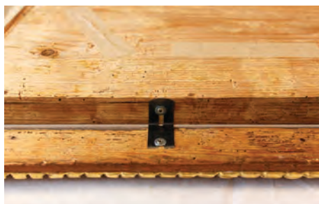
Fig. 25. Rectangular strap fastening on the sides for greater stability, preventing the box and frame from moving
