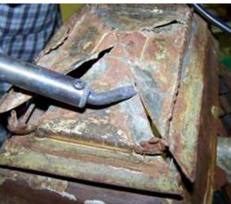
Fig. 18. Disassembling the birdcage roof using a soldering iron
